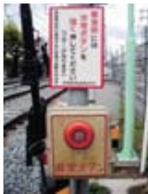
踏切支障報知装置 ▶
